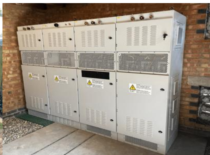
Installation with 3 off DGI-400 and neutral cabinet for Soft Open Point
